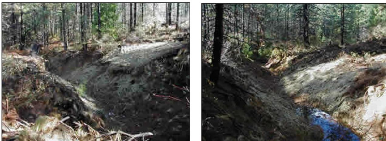
The situation was an ephemeral drainage line used during August, when the chance of measurable precipitation was minimal. The crossing was removed by September 1. There was no pipe or separator material used. Whole trees 250-600mm diameter breast height were used in the drainage channel. After the crossing was no longer needed, the material was removed with a heel-boom loader and processed at the landing. Standard erosion control measures were required.
