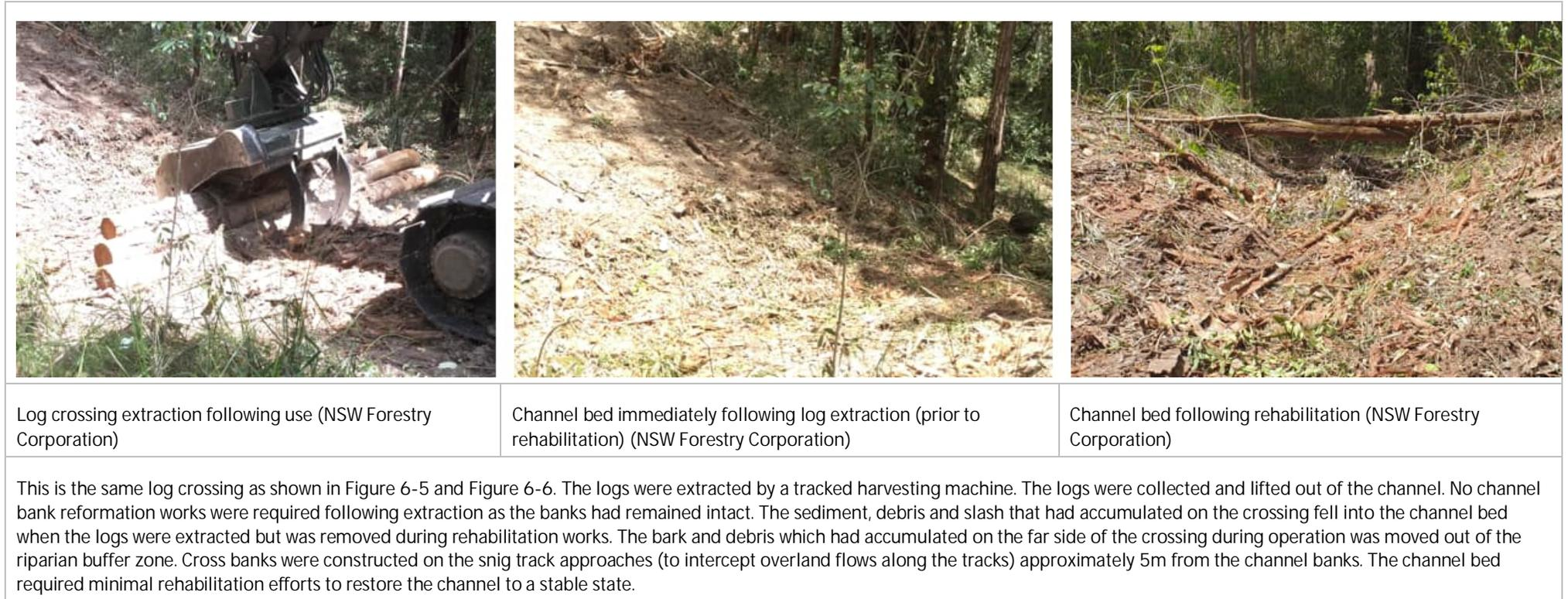
Figure 6-7 Temporary log crossing during extraction, prior to and following rehabilitation, Wauchope region, NSW. Source: NSW Forestry Corporation
