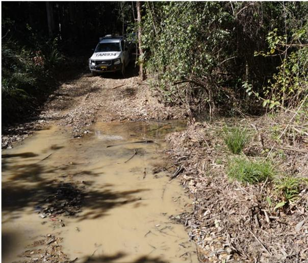
Causeway crossing in on-going use, with evidence of sediment generated following vehicle passage. Note that this is a road rather than temporary track crossing.
