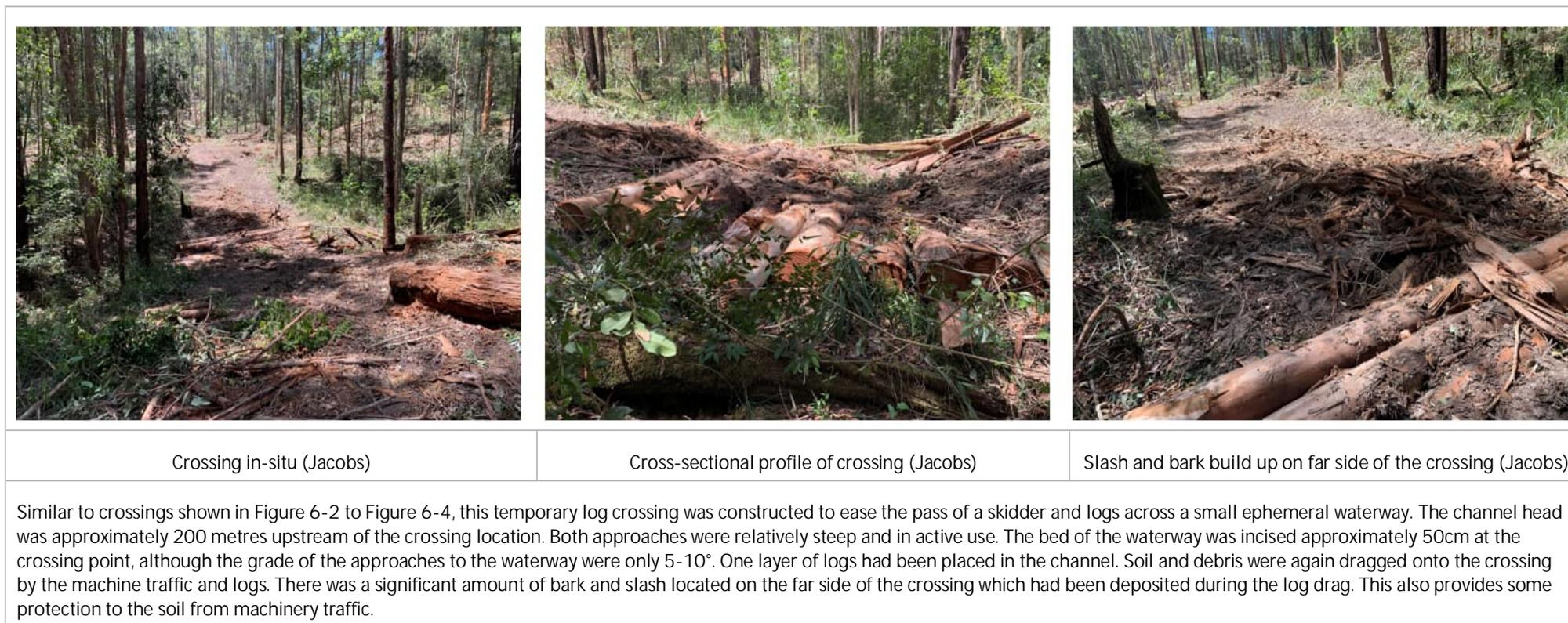
Figure 6-5 Temporary log crossing in-situ during second site visit, Wauchope region, NSW. Source: Jacobs
