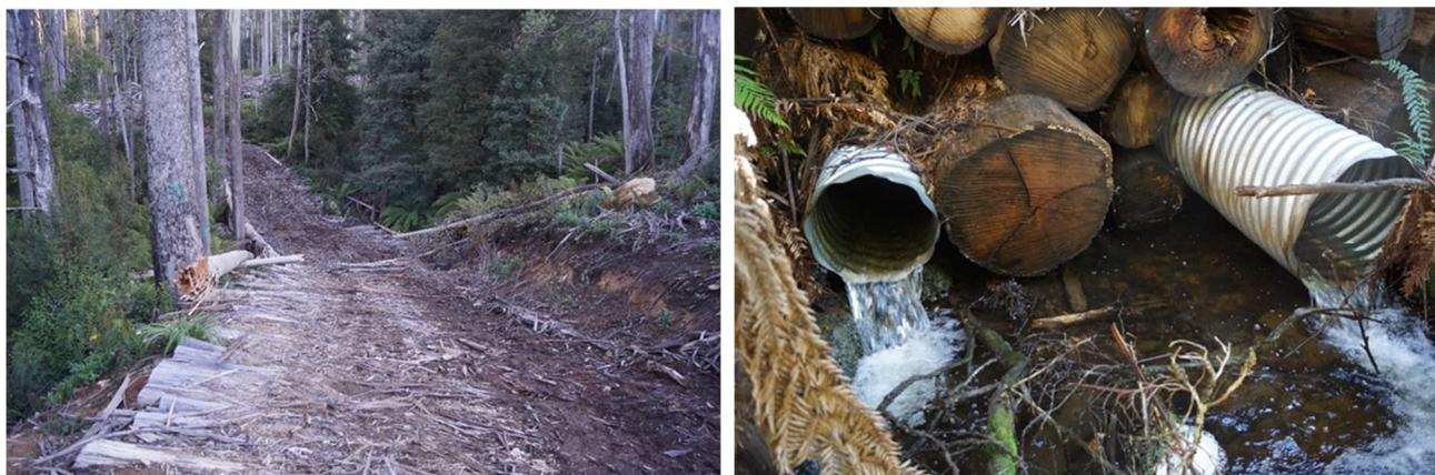
Figure 5-3. Temporary log crossing in use as a forwarding track across a permanent stream in tall, wet eucalypt forests in Victorian Central Highlands region. Source: Jacobs (2020).
